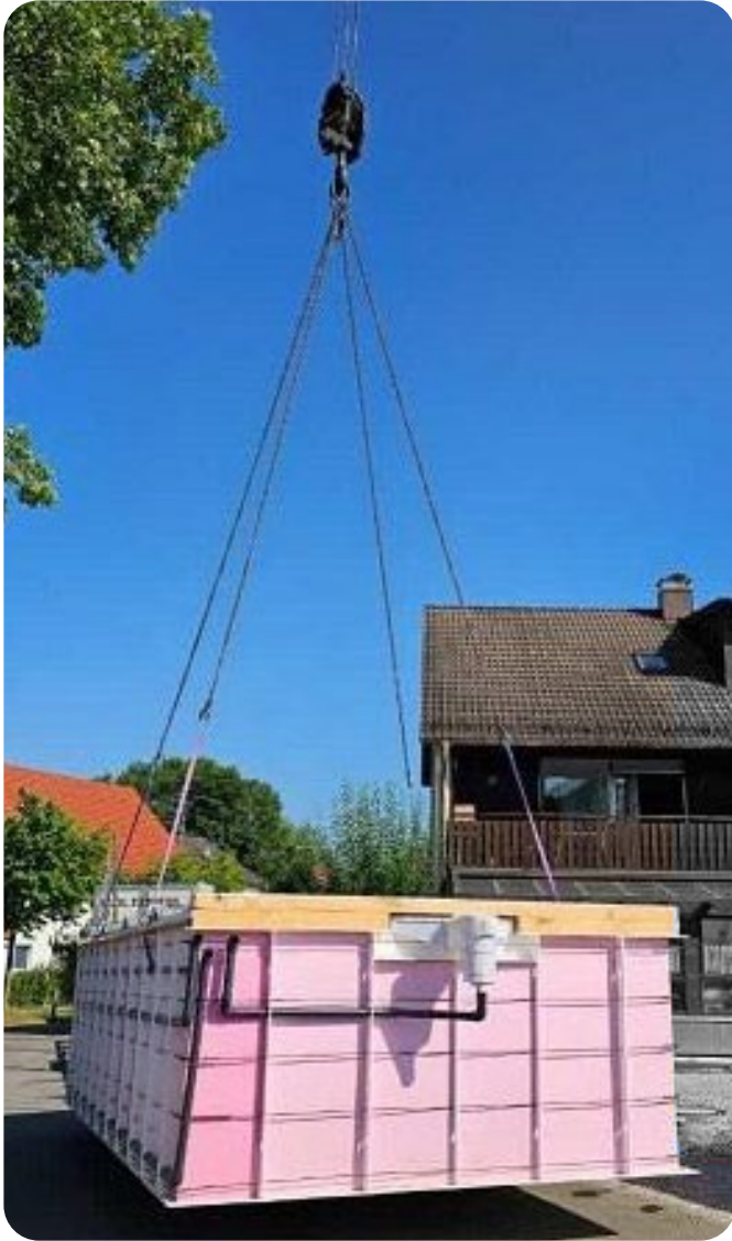
Lifting the pool in a horizontal position.
