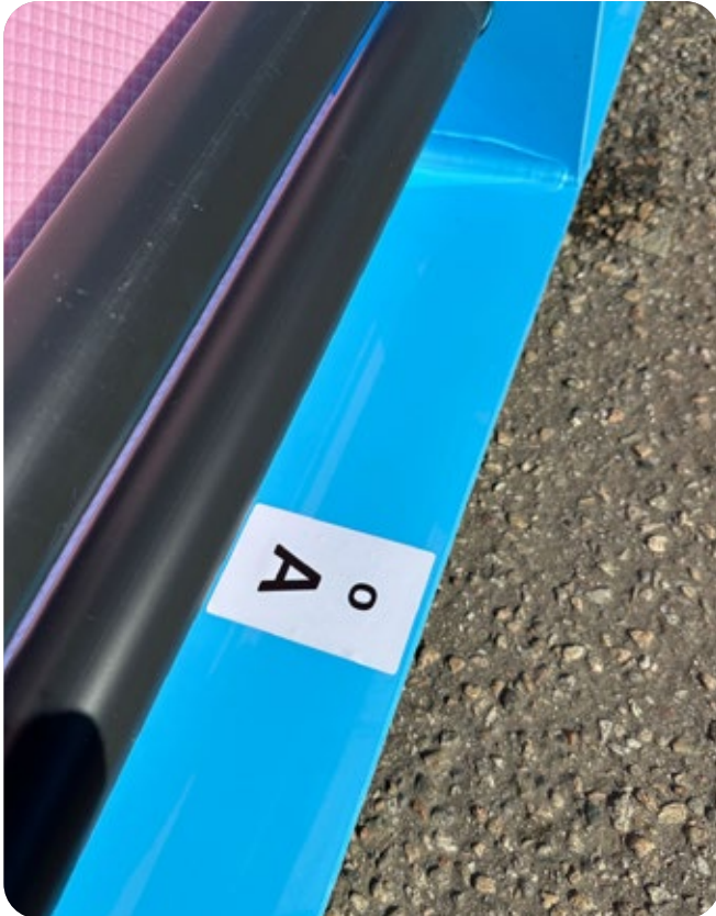
Marker indicating where to drill
